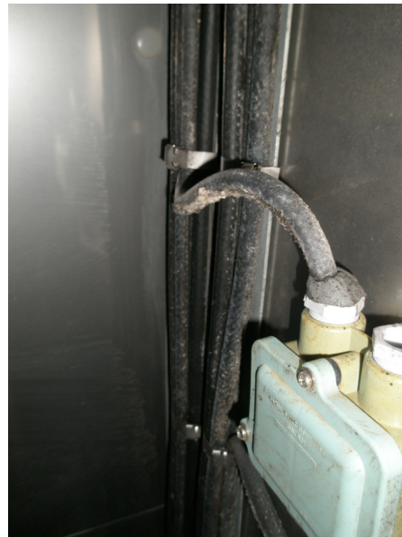
Heavy Mould on pipes and fittings could drop off into food
