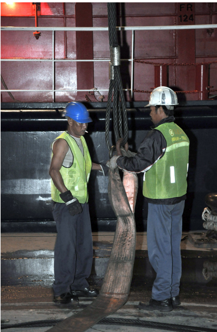
Shore Labour preparing a sling.
