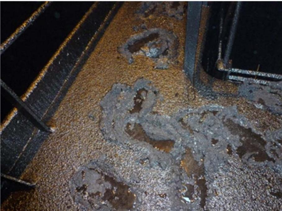
*Significant cargo ROB on tank floor, showing footsteps after inspection.*
