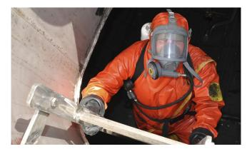
Accumulated pollution in the tank is also an issue, especially if a long time has passed since the last tank cleaning. If the pollution is considerable, it may contaminate the new fuel to a level where even the separator will have problems removing it. Lighter fuels will have a washing effect on the tanks, causing pollution to come loose over time and contaminate the fuel for a lengthy period to come.
