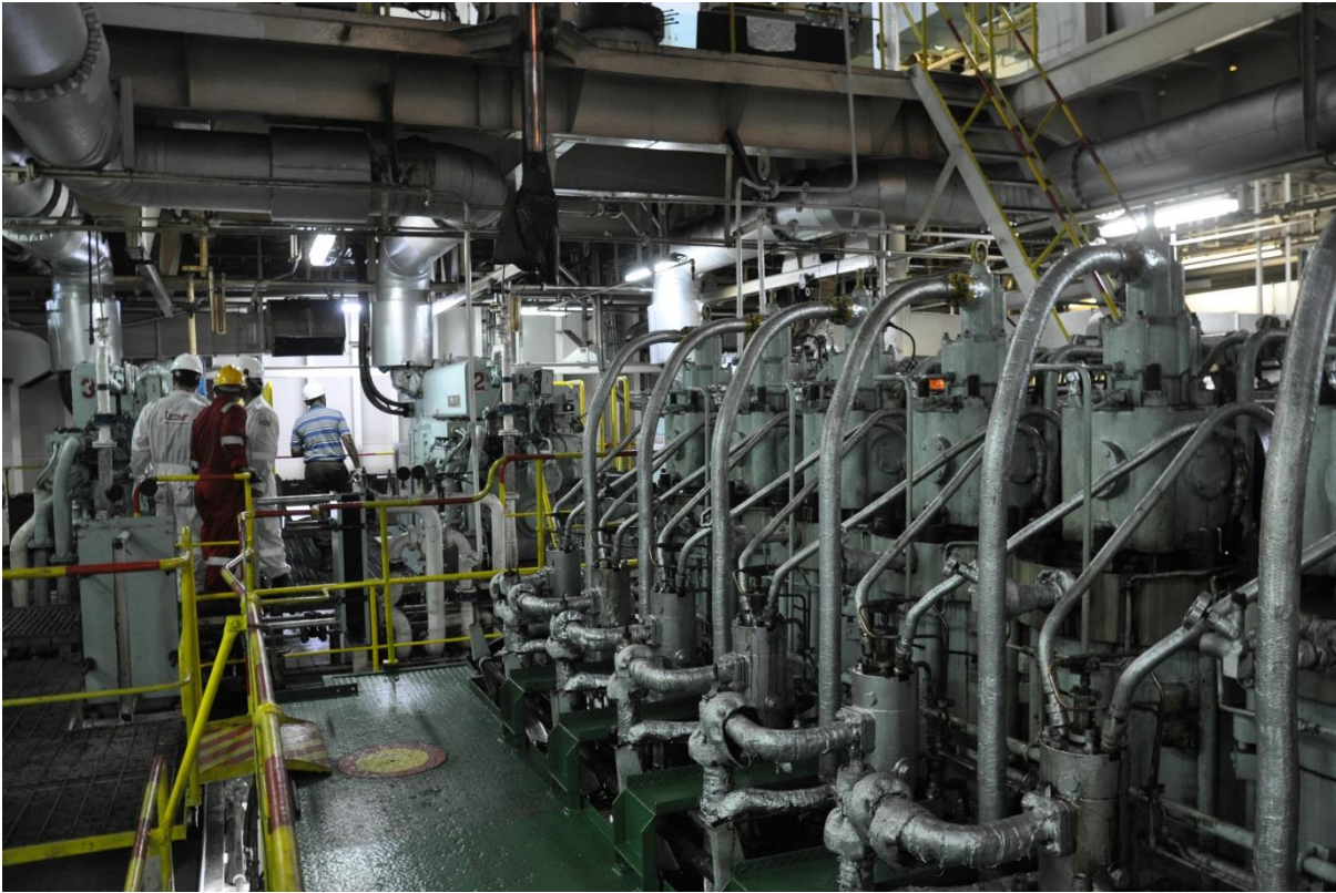
Engine Room Inspection
