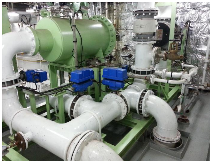
Ballast Water Treatment System on a vessel
